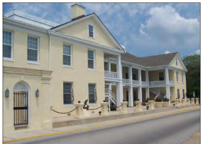
St. Francis Barracks.
