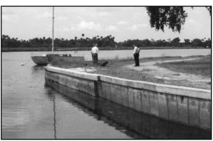
To the left is the seawall protecting the back face of Crystal River mound. A seawall is a structure separating land and water areas primarily to prevent erosion and other damage caused by wave action.
